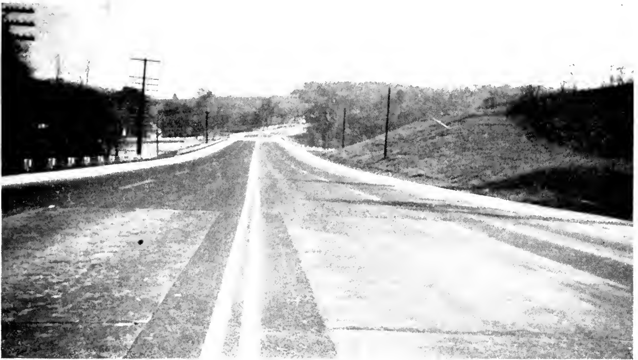
RELOCATION OF U.S. ROUTE 140—REISTERSTOWN TO WESTMINSTER. LOOKING SOUTH TOWARD BRIDGE OVER NORTH BRANCH OF PATAPSCO RIVER
